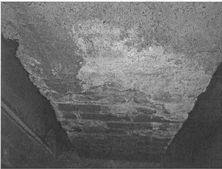
Photograph 7: View of the deteriorating chimney in the boiler area with efflorescence present, an indicator of elevated moisture content.
