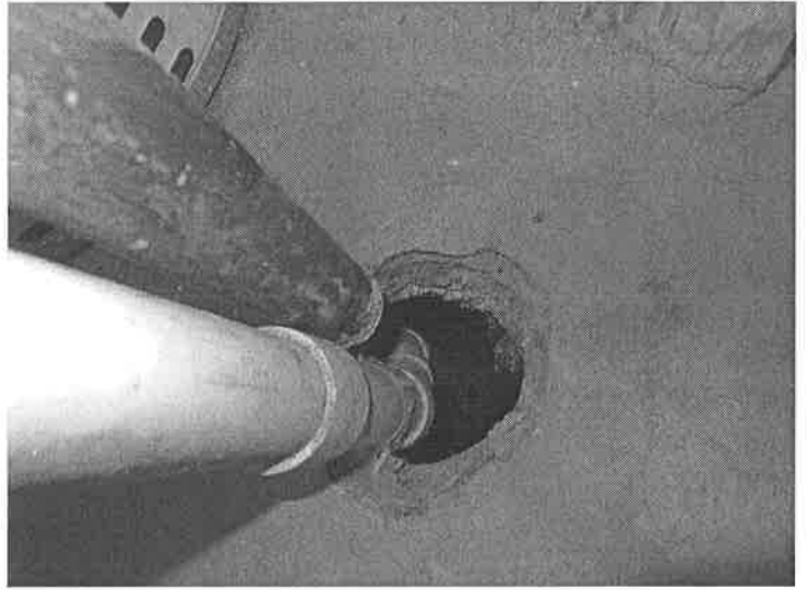
Photograph 6: View of a hole in the concrete flooring in the boiler area.
