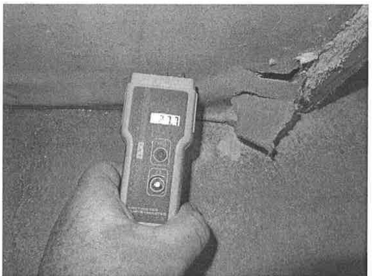
Photograph 4: View of elevated moisture reading (27.7%) in the deteriorating gypsum board on the south wall of the boiler area.
