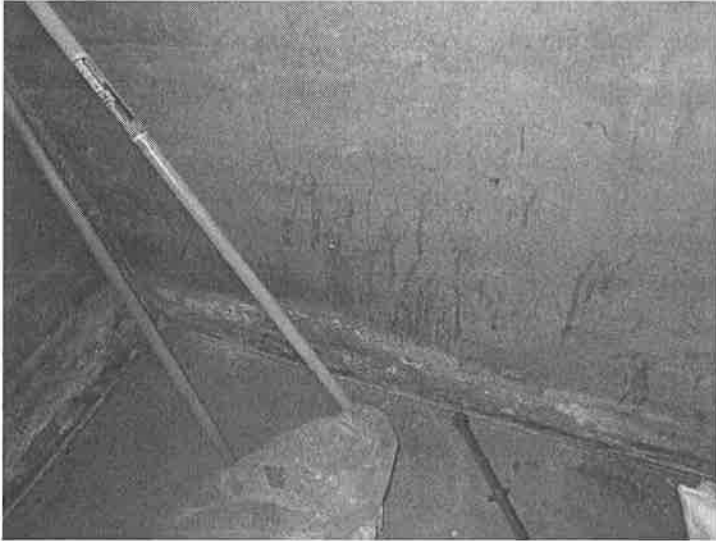
Photograph 5: View of water staining on the lower north concrete wall in the boiler area.
